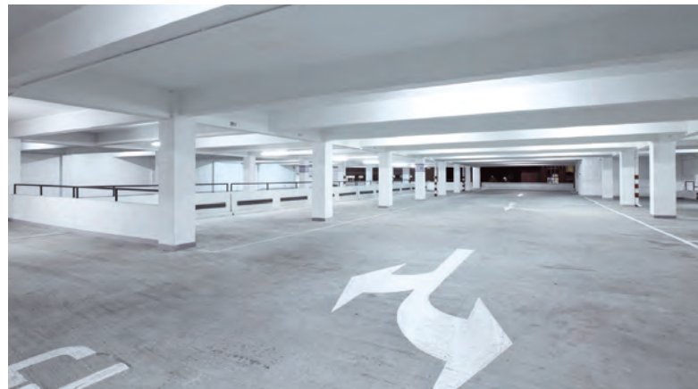
UNDERGROUND CAR PARKS
